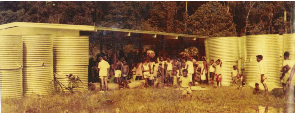
The Kapore Community Centre 1968 with water tanks ready for distribution to each smallholder block in the oil palm subdivision
